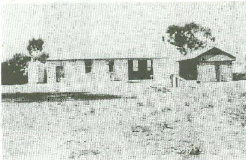
Cadell Primary — Circa 1930's Note condition of playing surface.
